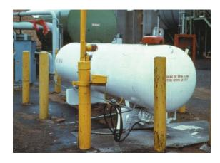
Propane tank used to refill the forklift LPG tank is protected against vehicle damage by heavy posts and must be well ventilated and not near any ignition sources.
