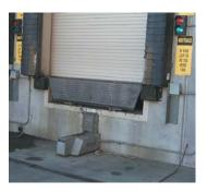
Dock mounted vehicle restraint clamps to a bar under the truck.
