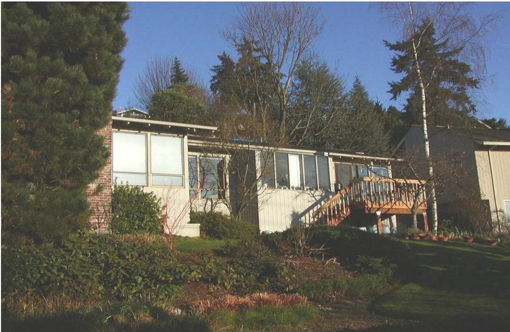
Photo 4: A view of the residence where the incident occurred from below, on the opposite side of the house from the truck and plank.
