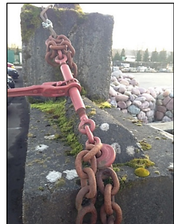
Photo 4. Ratchet mechanism for tightening wall cable
