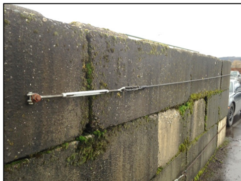
Photo 5. Steel cable bolted into side of ecology block wall
