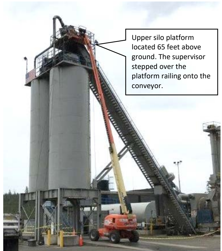
Photo 1: Asphalt storage silos and the drag slat conveyor down which the supervisor slid and fell while performing maintenance on the upper part of the conveyor. The two workers used the aerial lift to access the silo platforms.
