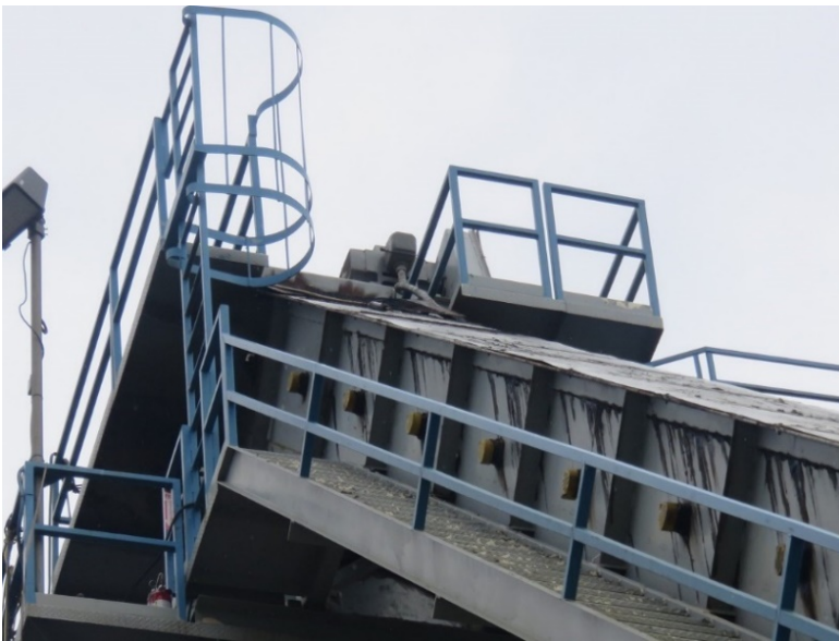
Photo 4: Rails on platforms that employees climbed over to access the conveyor gearbox. The supervisor climbed over the rails on the upper left side of this photo.
