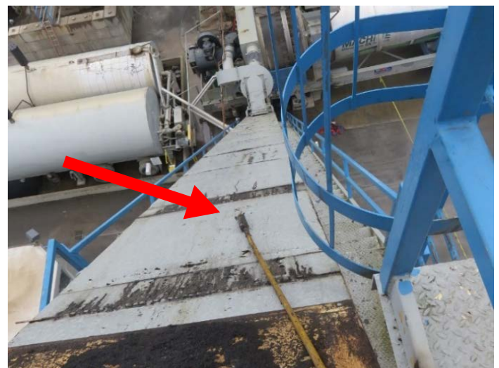
Photo 9: The conveyor cover down which the supervisor slid feet first, face down and then fell to the concrete slab below. Arrow shows the airline and the pneumatic chisel that the supervisor was preparing to use.
