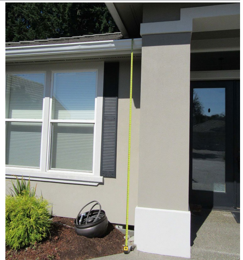
Figure 1: The tape measure shows where the ladder was set up. One foot was on the mulch, the other foot was on concrete.
