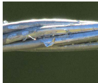
Cross cable with damage possibly caused by being snagged on bolt on top of harvester.
