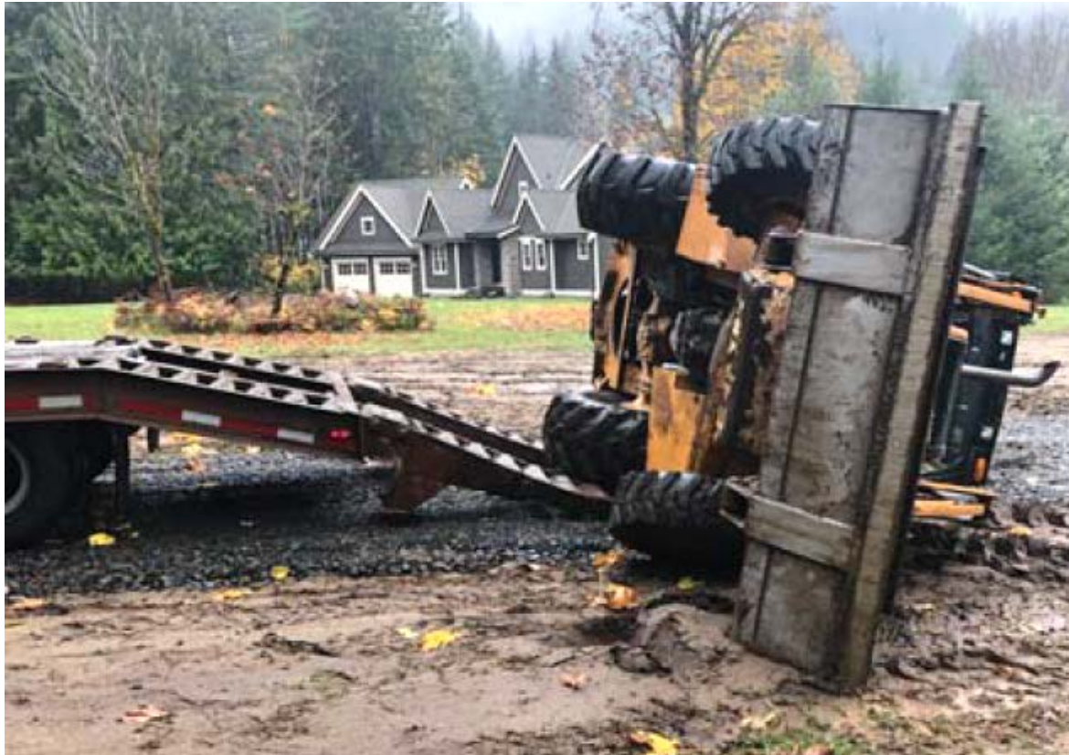
Photo 2. Backhoe rolled over on its side and trailer ramps.
