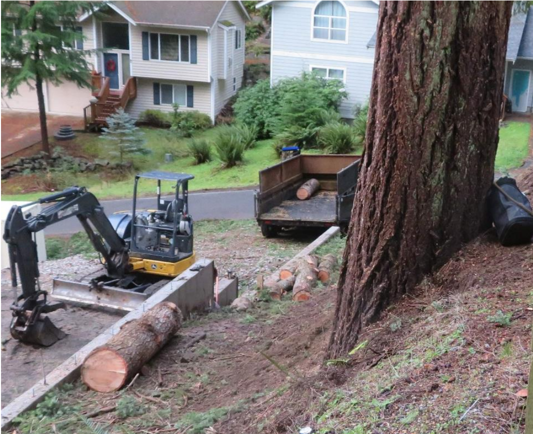
Photo 5. Incident scene with 330-pound section at bottom of embankment down which the worker fell.
