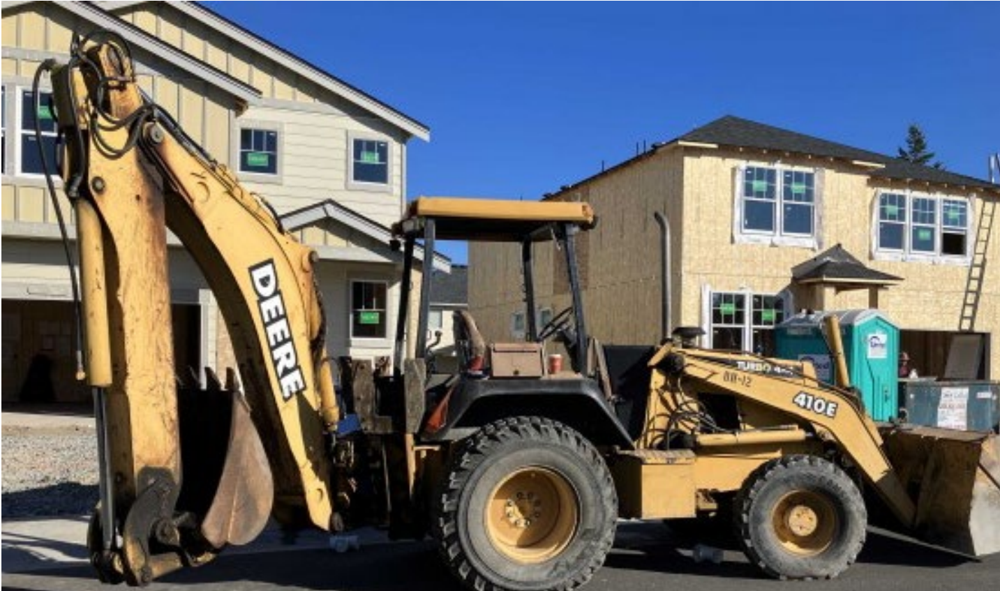
Photo 1. Backhoe loader at the incident scene
