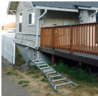
Unsecured top half of ladder resting on the grass surface.
