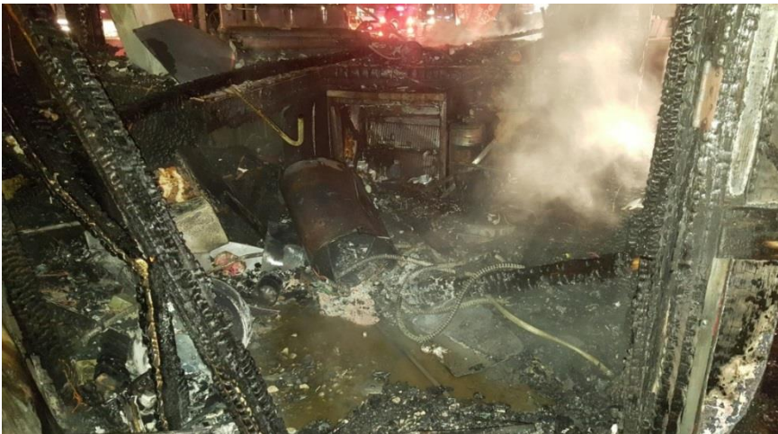
Photo 2: The coffee stand interior after the fire.
