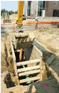
View from excavator cab. The spotter was in the trench to the right in the operator's blind spot.
