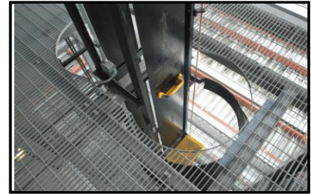
View of manlift coming up to landing
