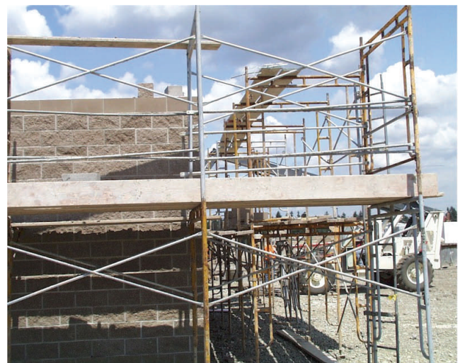
Scaffold properly guarded
