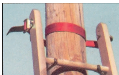
Make sure the ladder is secured to prevent it from slipping, moving, or falling over.
