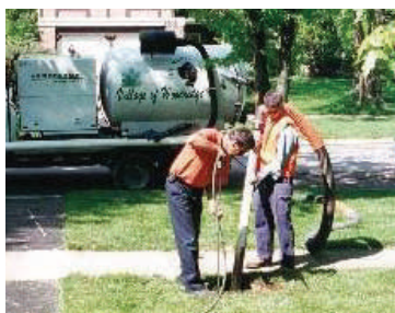
Hydro excavation machine
