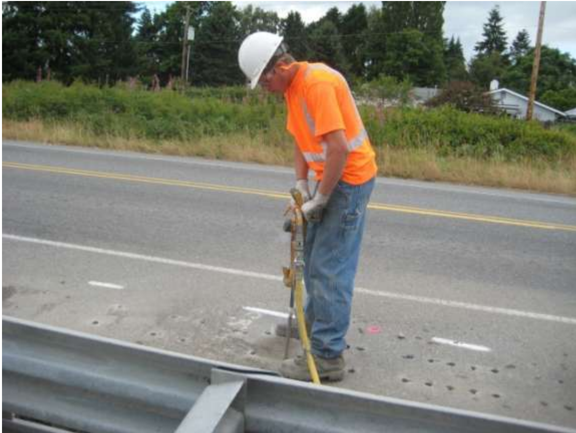
Figure 1: Dale Aamot drilling anchor holes for temporary impact attenuators along SR 20.
