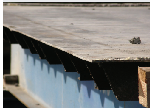
Metal edges can present a deadly risk to lifelines and lives. The edge on the steel plate shown above cut a worker's steel cable lifeline shown below.
