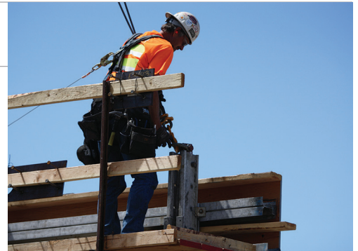
Lifelines anchored horizontally necessitate extra safety precautions when working near metal or concrete edges along decking, floors, roofs, platforms, formwork, and other surfaces.
