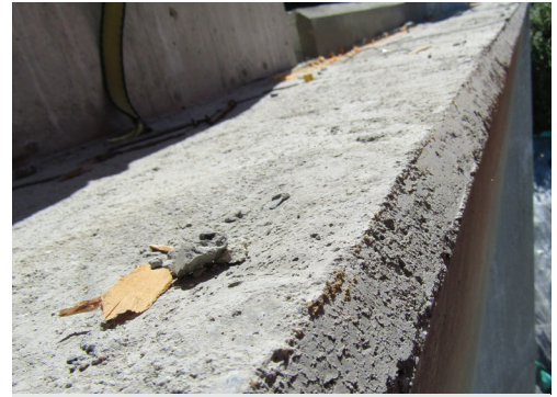
The exposed edges (shown above) cut a worker's nylon webbing lifeline (shown below) during a fatal fall.
