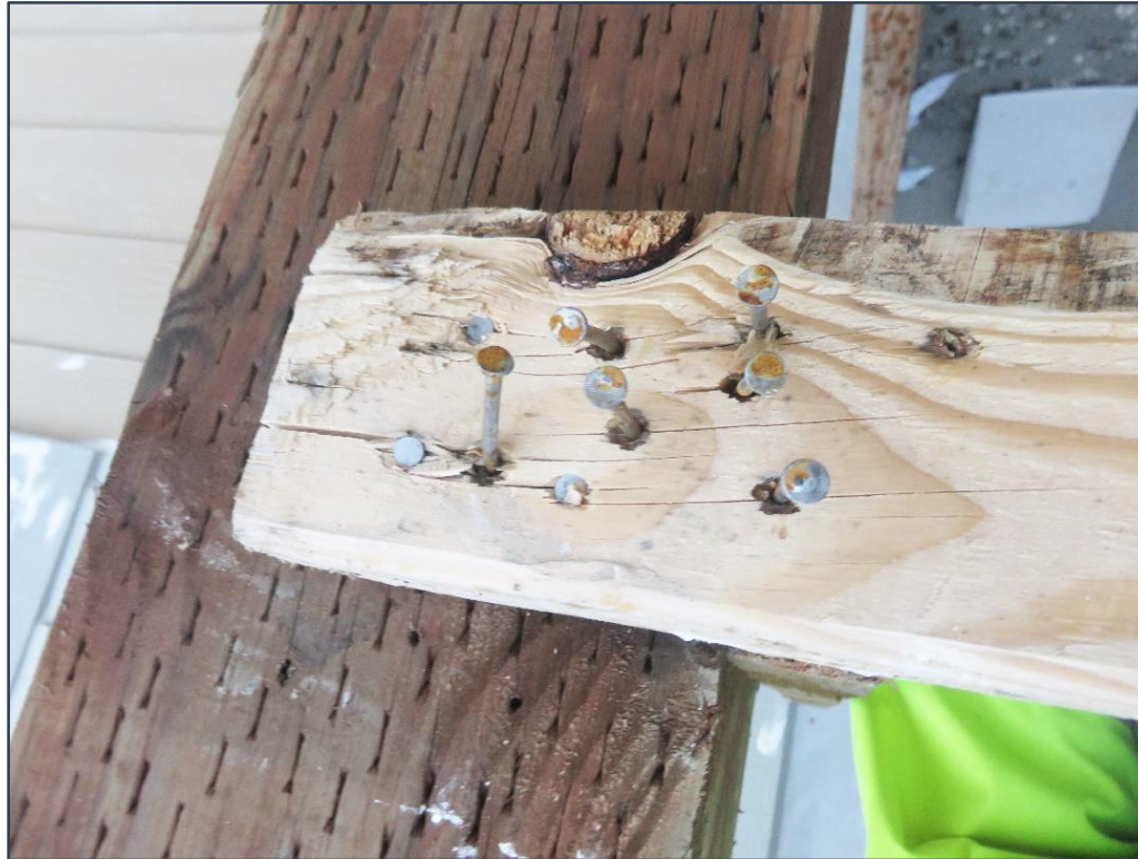
Photo 5. Railing (not incident railing) at job site showing multiple nails. Workers needed to remove railings to install moisture barriers on the building.
