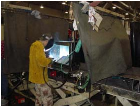
A scissor table helps this welder to work in a more upright position.
