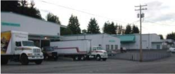
Figure 1. Jennings Distributing receiving docks.
