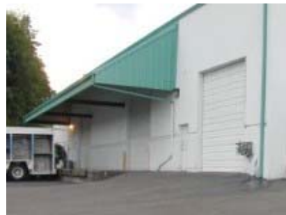
Figure 15b. Wine loading dock ramp.
