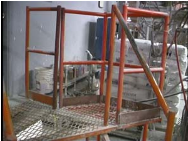
The old way: Platform extension to improve access
