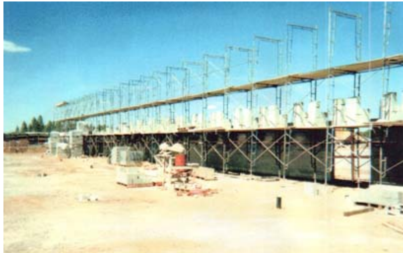
Welded tubular frame scaffolding
