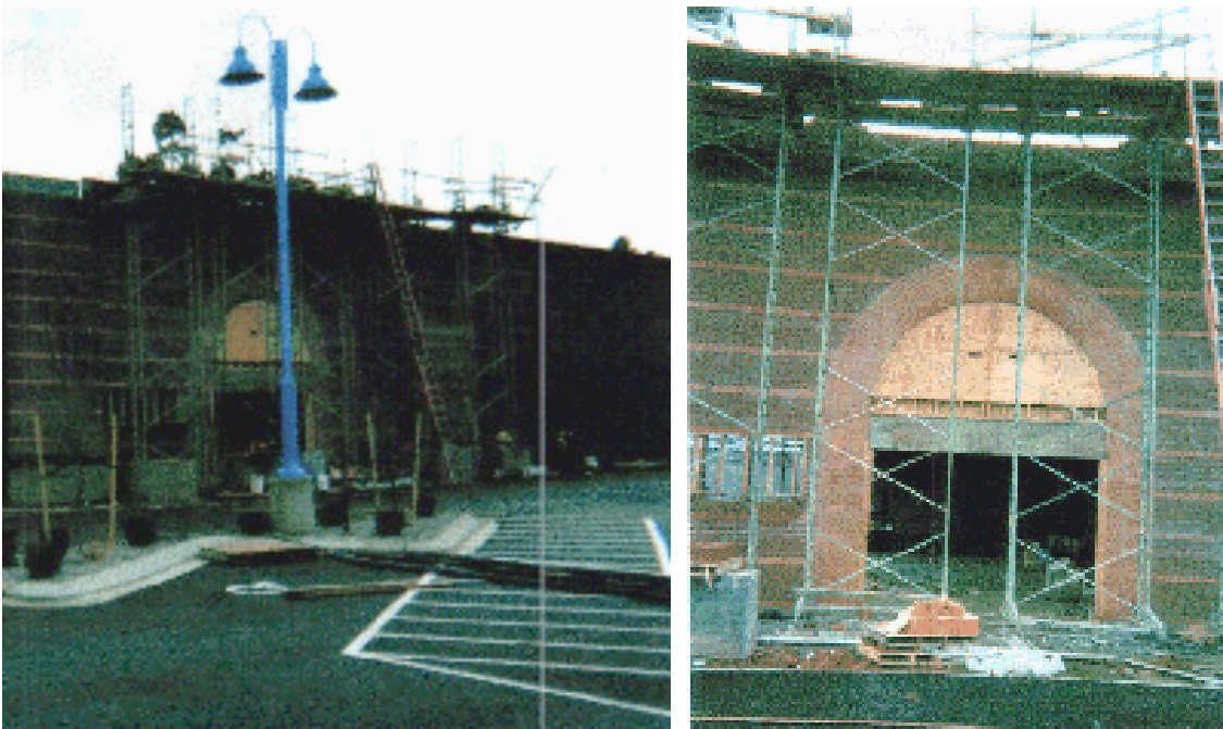
Two examples of the manual crank tower scaffolding (Non-Stop)
