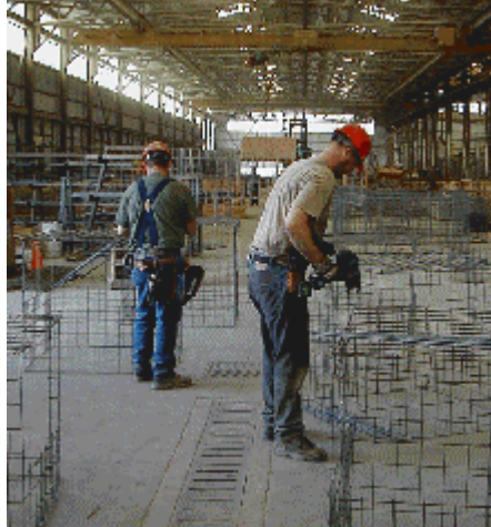
Figure 1. Utility Vault workers using rebar tiers on reinforcement mesh and rods.
