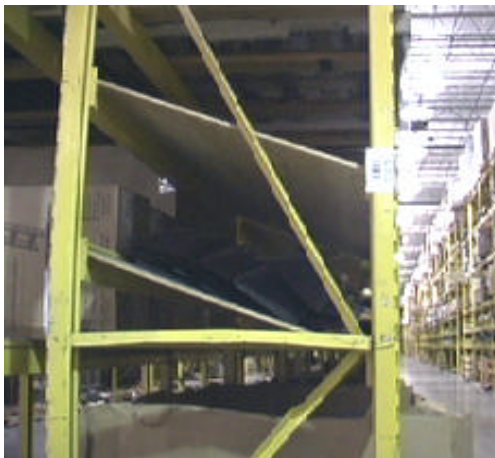
Storage bins are constructed with a floor slanting forward easing access for both Stockers and Order Fillers.
