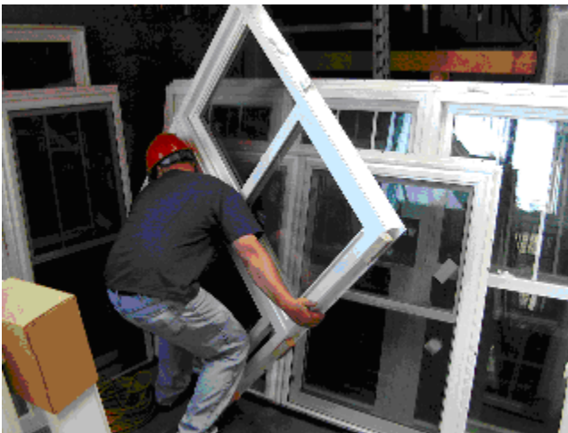
Figure 3. Lifting window assemblies.
