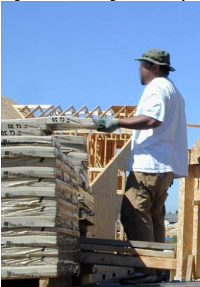
a) Lifted off pallet (top of pallet) (bundle slid off top of pallet)
