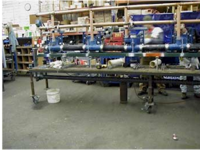
Figure 4. Pre-assembly of a plumbing sub-system on a portable, rolling framework.
