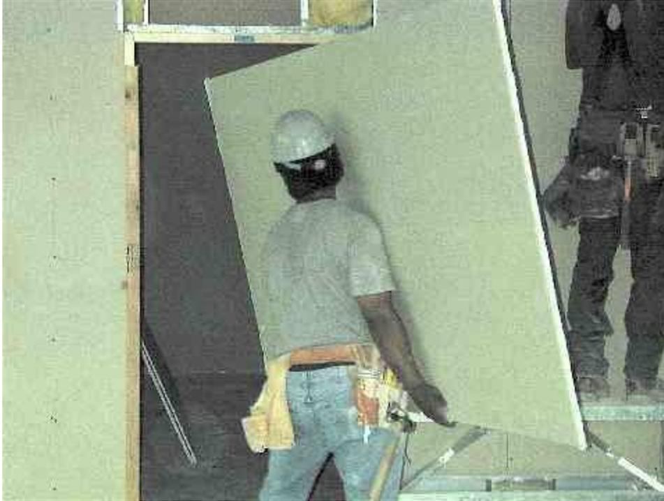
**Figure 1.** Lifting heavy wallboard panels for installation.
