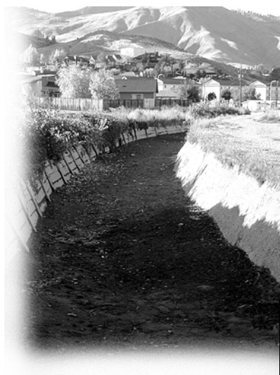
Irrigation ditches, such as this, contain hidden dangers.
