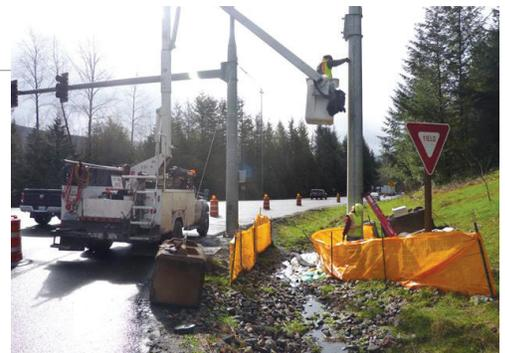
Traffic control measures, like the barrier cones used in this picture, can prevent motor vehicles from coming into contact with elevating work platform.
