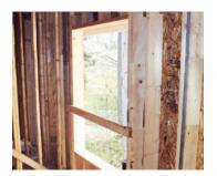
Guardrails are required across window openings that have sill heights less than 39 inches.
