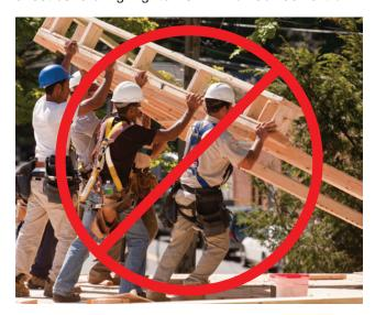
Workers are exposed to falls while raising a wall without using fall protection. Workers will also be exposed to falls through the unguarded wall opening once the wall is anchored in place.
