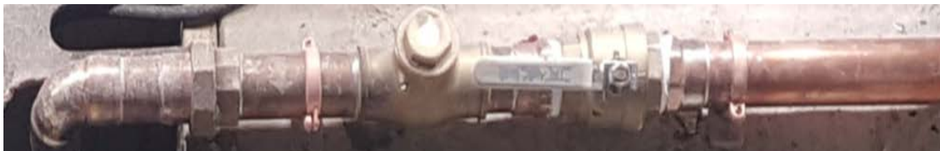
Figure 1 Suggested plumbing fittings and connections: union; check valve; shut-off valve.
