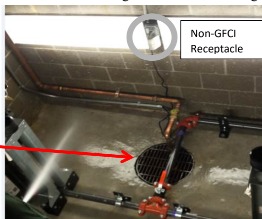
Figure 2 Non-GFCI receptacle and open grate cover (round or square as applicable).
