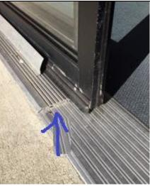
Arrow shows difference between old threshold and new, lower threshold
