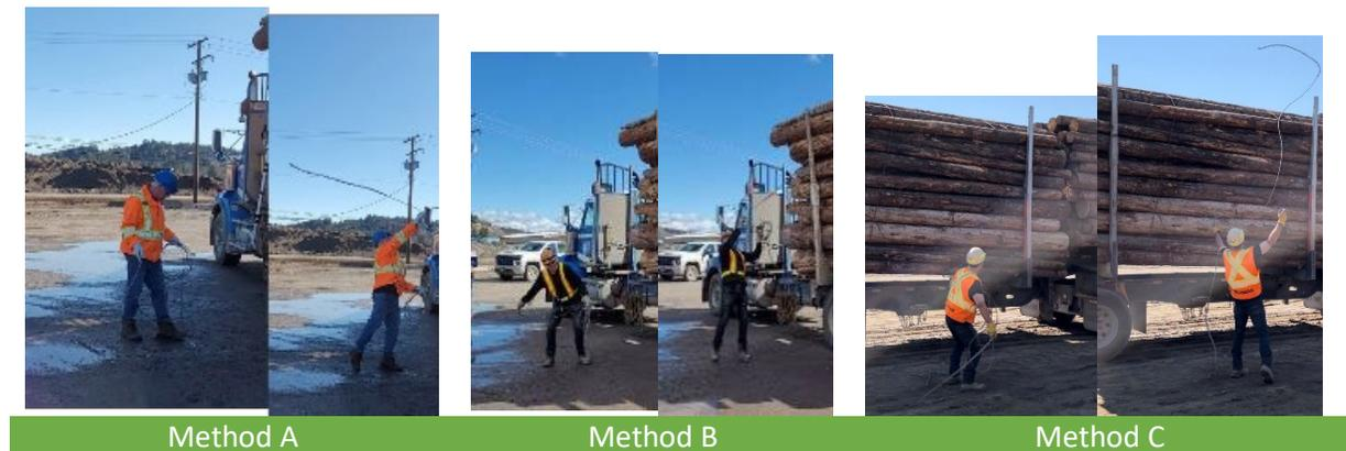
Figure 9. Alternative throwing methods using 5/16” steel wrappers.
