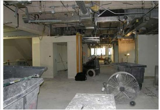
Running just one propane-powered machine in a poorly ventilated space can lead to carbon monoxide poisoning, even in larger spaces like this one.
