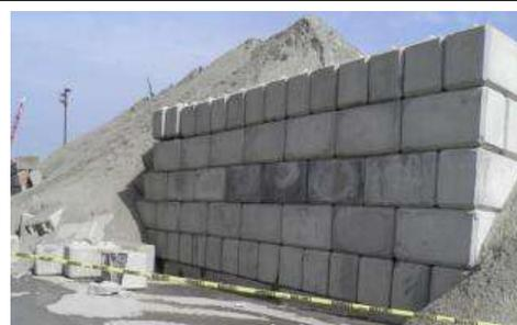
These walls can tumble down. Too much bulk material exerts enough sideways force to cause concrete blocks or whole sections of walls to suddenly collapse.
