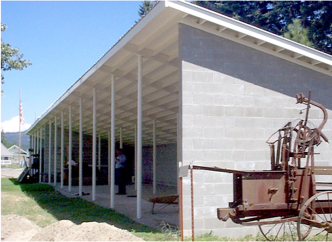
Photo #1. The exterior of the building under construction.
