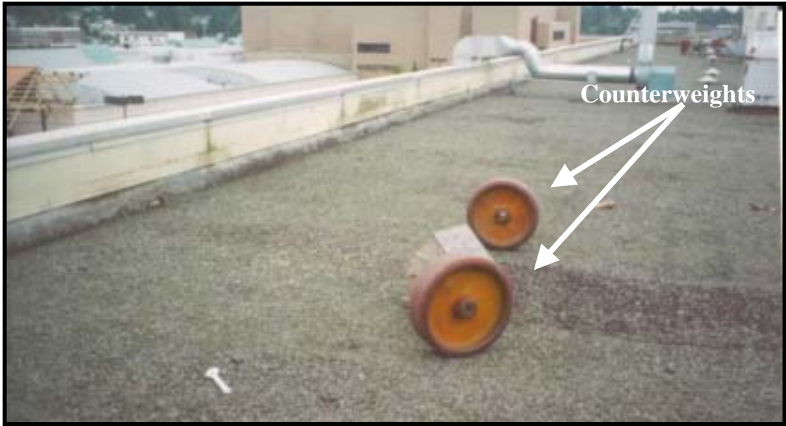
Figure 3. Roof top from where victim fell and counterweights.
