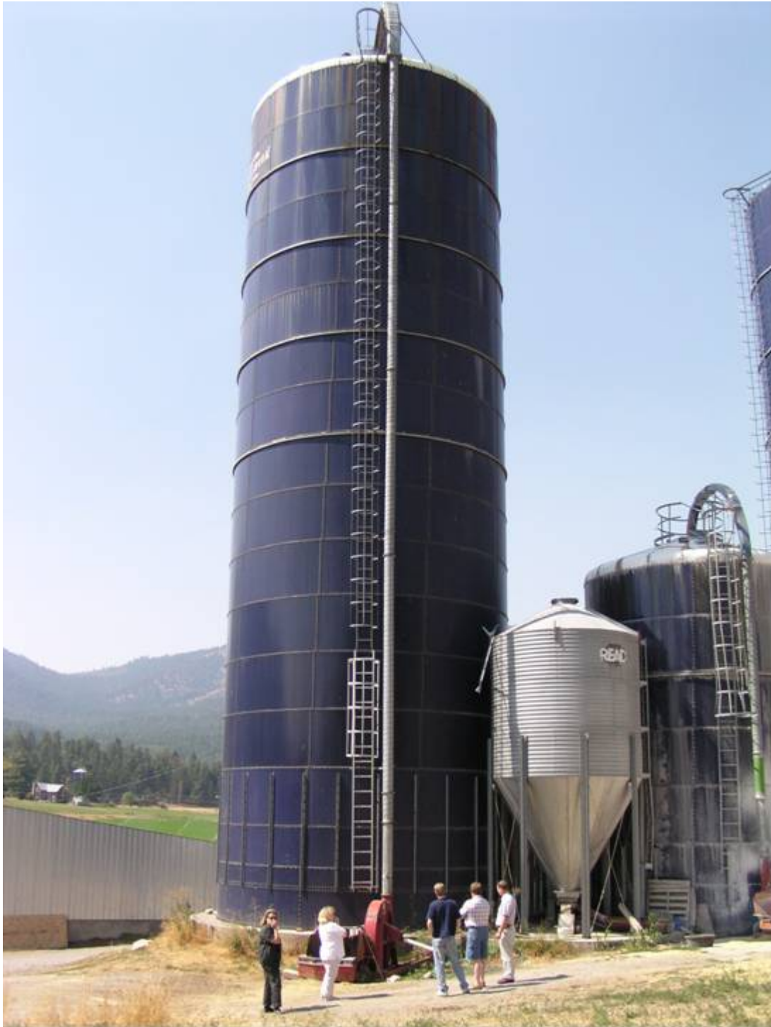
Photograph 3. A view of the silo from ground-level.
