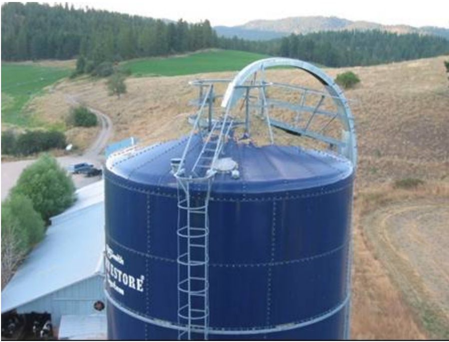
Photograph 1. A view of the top of the silo with ladder cage and chute extended after filling.
