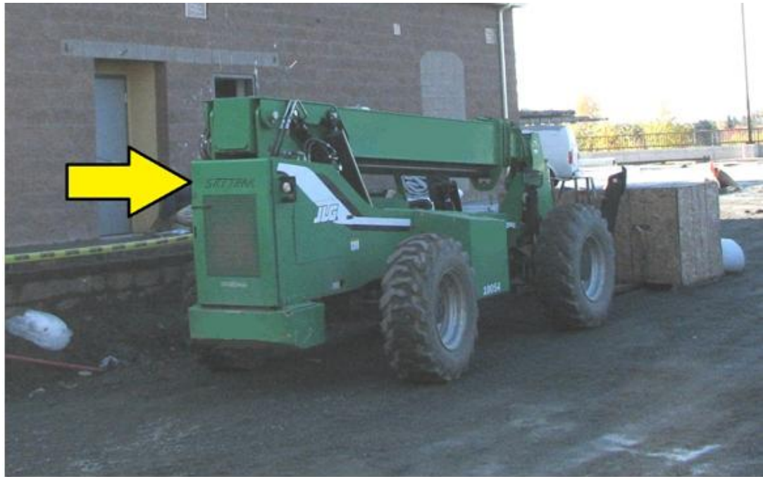
Photo 2: Telehandler used to raise the skip box
