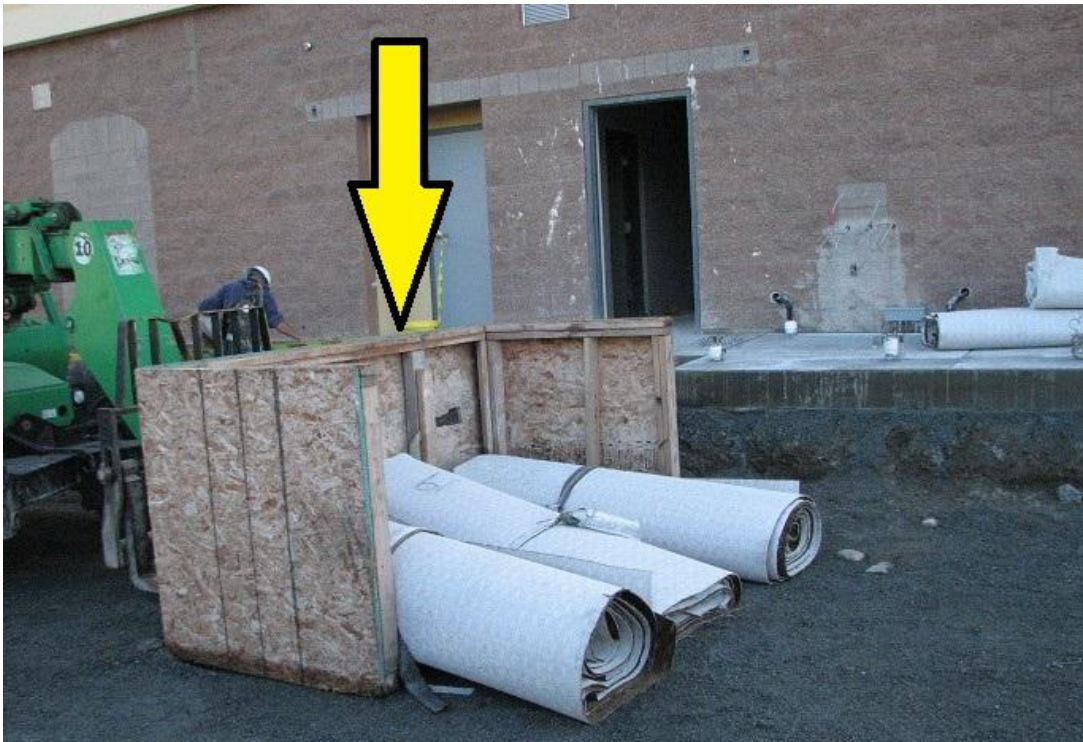
Photo 1: Three-sided skip box used to elevate carpet rolls to window
