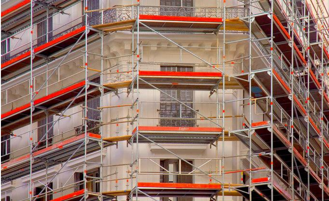
Photo 7: Example of scaffolding platform
