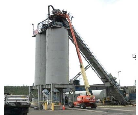
Asphalt storage silos and the drag slat conveyor down which the supervisor slid and fell while performing maintenance on the upper part of the conveyor.
