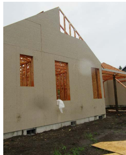
Side of house where framer placed extension ladder on soft dirt. As he was climbing, it shifted and he fell eight feet.
