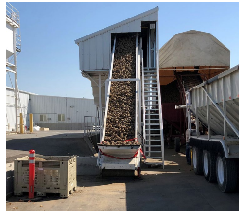
Elevator conveyor overloaded with potatoes, which led to the jam.
