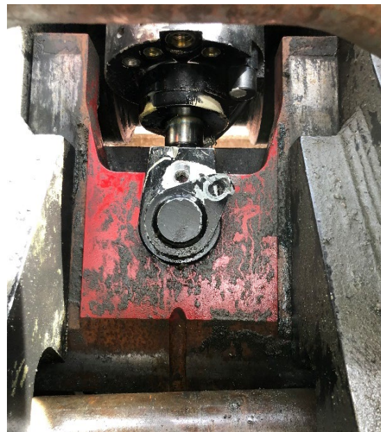
The wedge lock of the quick coupler that crushed the worker's fingers.
