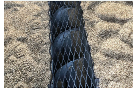
Incident 2: Floor auger with the metal grate cover. The grate could be removed and replaced with steel plates that a loader could drive over.
