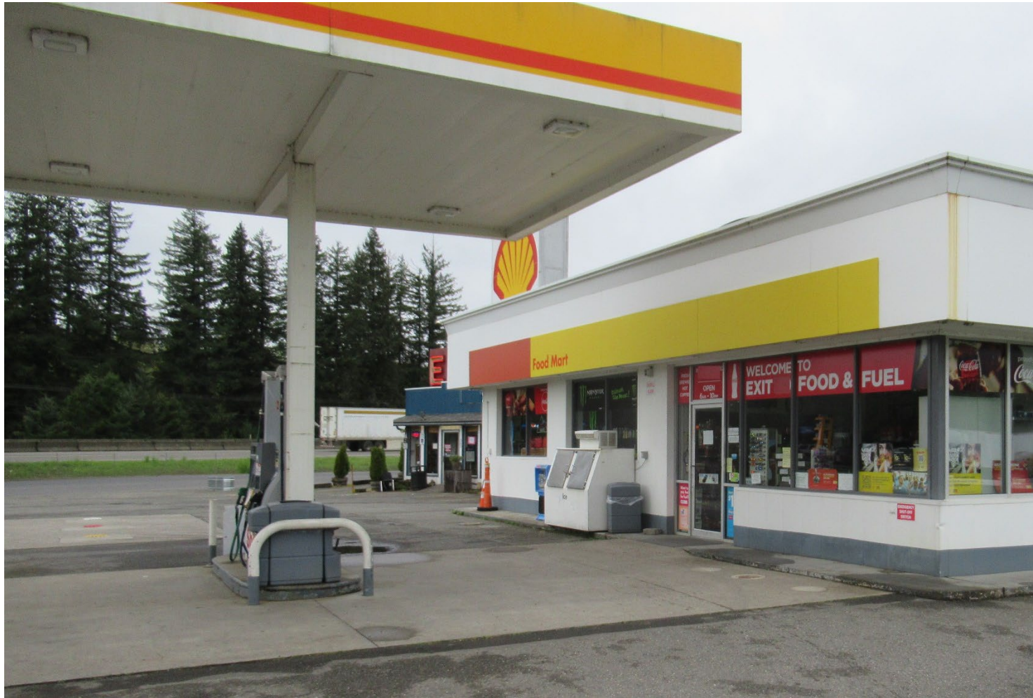
Photo 2. Closer view of gas station convenience store.
