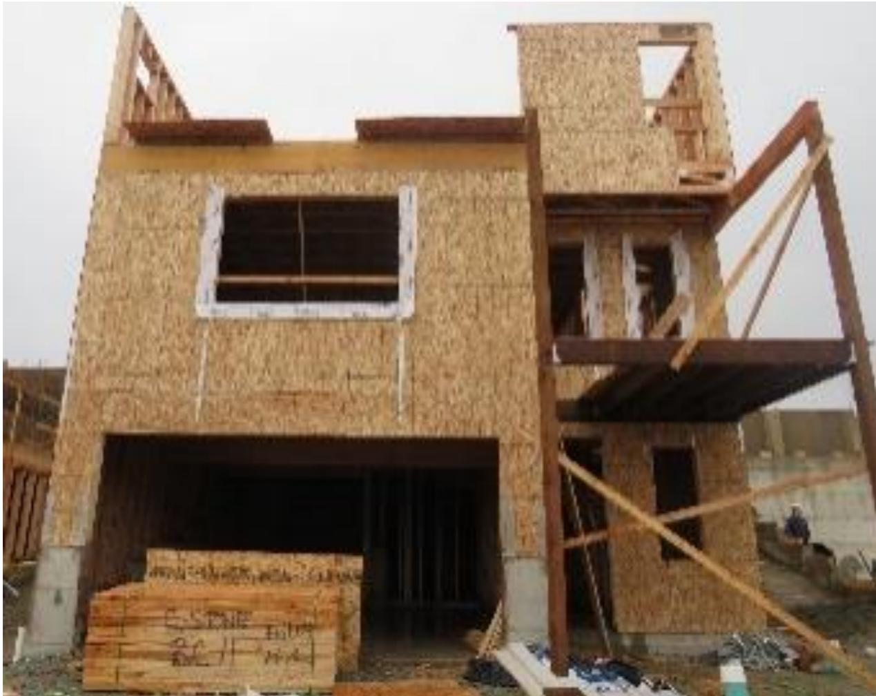
**Photo 1.** Open-sided upper floor where guardrails were removed.
