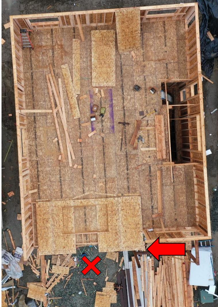
**Photo 3.** Aerial view of upper floor with arrow showing wall sheathing extending over unprotected edge.
