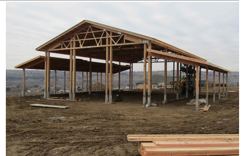
Figure 1: The pole barn under construction.
