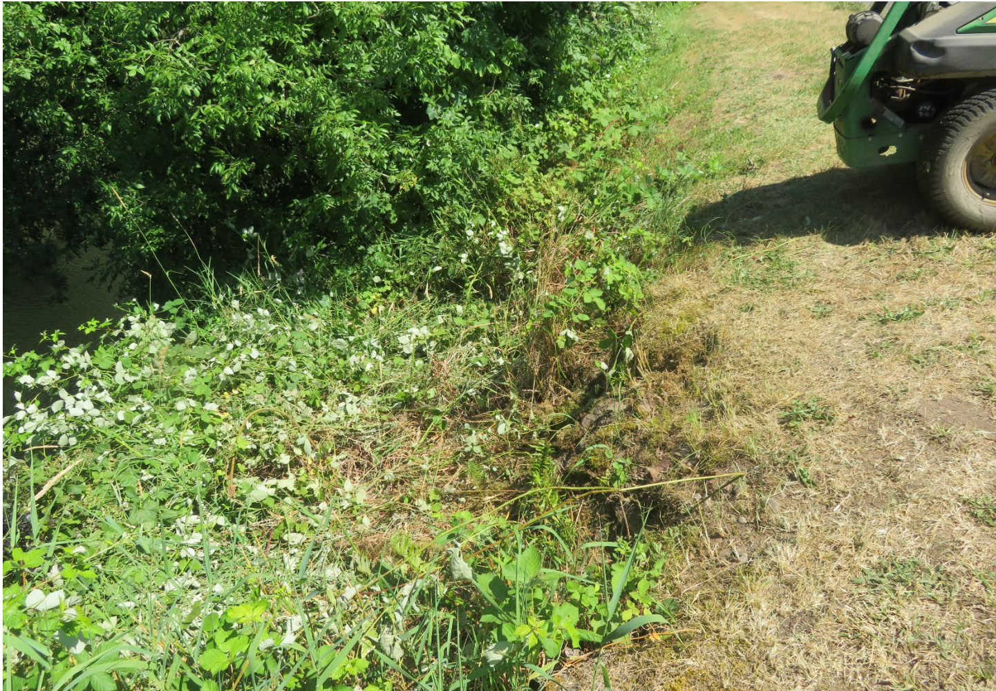
Photo 5. Eroded drop off on side of inner slope where mower rolled over.
